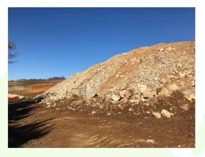
No stabilization measures applied to stockpile. No temporary silt fence.
