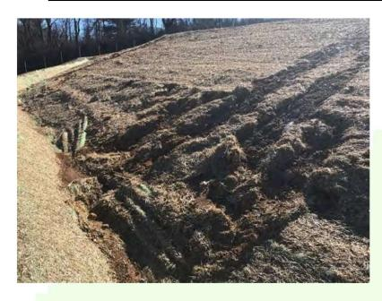
Erosion on slope above Ditch 5-3 East resulted in accumulation of sediment, decreasing capacity of ditch. Ditch not cleaned out.
