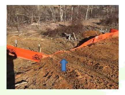
Silt fence behind Basin 3-3 not maintained in an effective operating condition.
