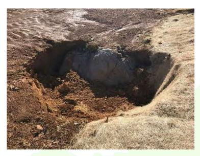
Sinkhole in Basin 3-3. Basin not maintained to hold the required wet volume per the Erosion and Sediment Control Regulations and the approved plan.
